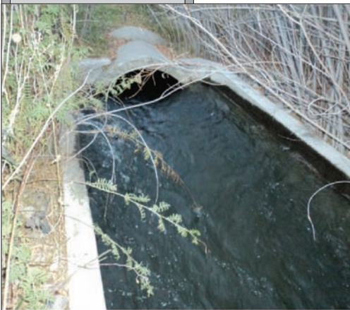
Figure 9. Diversion to Ground Water Recharge by Snake River Valley Irrigation District November 4, 2014
