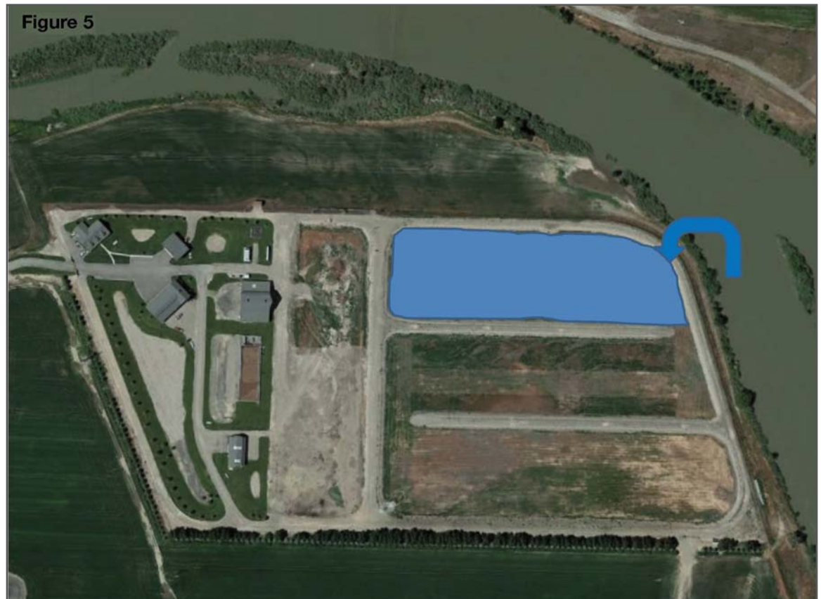
Figure 5. Recharge from Snake River into ponds that are not hydraulically connected to the river
